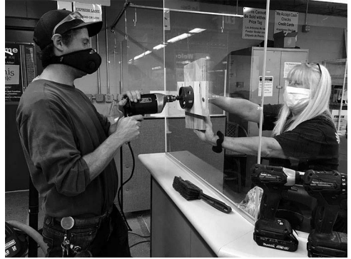
Installing plexiglass shields
